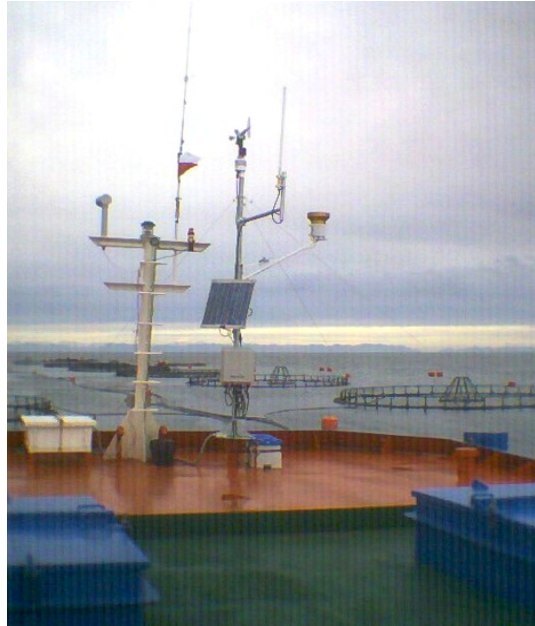
A monitoring station near sea cages in Chile
